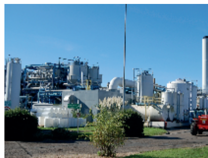
High Temperature Incineration, Hampshire
